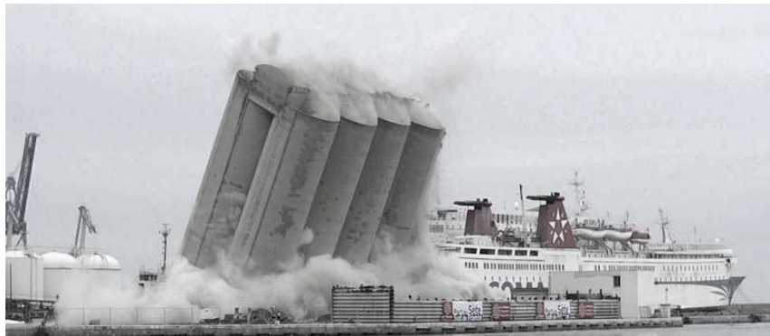
Picture 8.38. Tearing Down Silos
